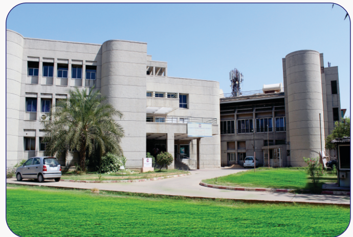
GTU - School of Pharmacy, Gandhinagar
